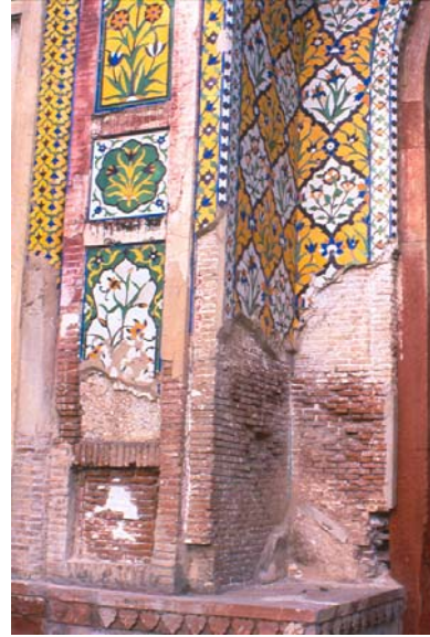
Figure 3: Eastern Gateway – tile work
